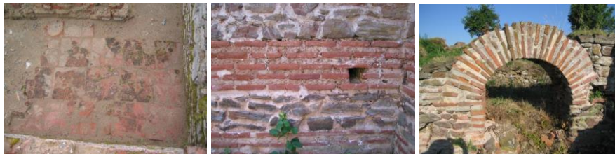
Fig. 5 Usage of bricks for floor tiles and wall construction at an early Byzantine site, Iustiniana Prima (6 th century) in Serbia. Photo A.Momčilović Petronijević and Č. Vasić
