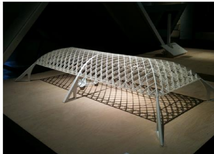
Fig. 2 Model of structure Orvieto hangar from Pier Luigi Nervi 7 (Source: O. Popović Larsen 2014)
