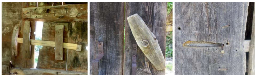
Fig. 10 Door locking mechanisms (photo I. Đorđević)
