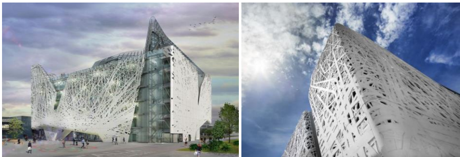
Fig. 11 a) The pavilion, the city of Milan, Italy for Expo 2015 [32], b) The pavilion, Milan, Italy for Expo 2015 –the part of the photocatalytic façade [32].
