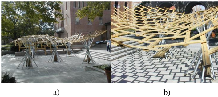
Fig. 6 Pavilion of the Forest Park: the whole structure 6 (Source: Gherardini et al. 2017)
