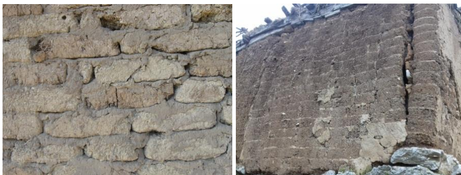
Fig. 3 Adobe on the buildings of vernacular architecture in Serbia. Photo A. Momčilović Petronijević.
