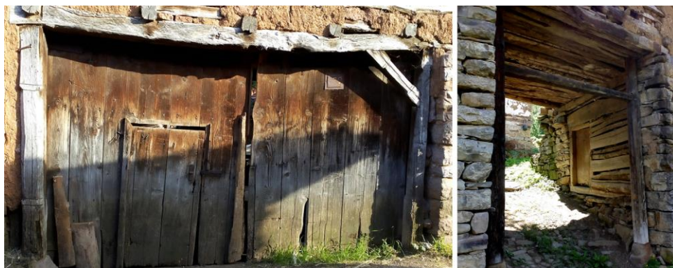
Fig. 4 Pedestran entrance obtained by cutting in the great gate wing (photo I. Đorđević)
