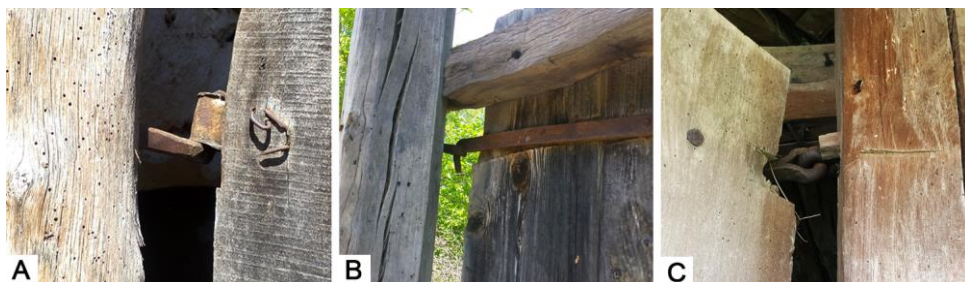
Fig. 9 Gate wing mounting (photo I. Đorđević)
