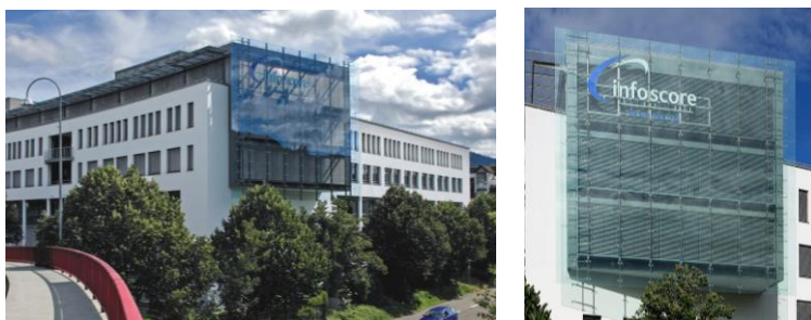
Fig 4. a) Infoscore office building, Baden-Baden, Germany [18] b) Infoscore office building, glass façade detail [19]
