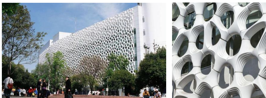
Fig. 10 The hospital building called the Torre de Especialidades, Mexico City [30, 31].
