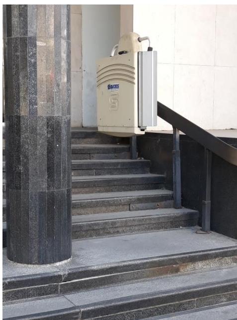
Fig. 2 Main Post Office building (wheelchair lifting platform has never been operational) (Photo: Branka Protić – Gava)
