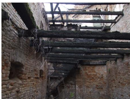
Fig. 7 Photograph of the interior of Salamon Halbrohr's barn, built in 1869. (photograph author: Viktorija Aladžić)
