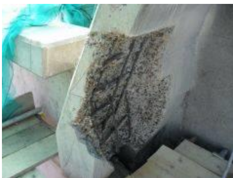
Fig. 6 Selective removal of deteriorated concrete
