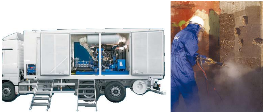
Fig. 11 Mobile equipment and concrete removal with hand-held water jet tools
