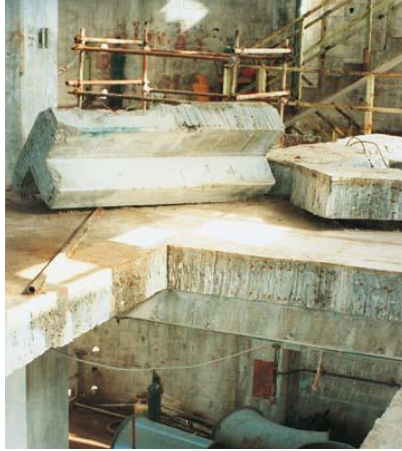
Fig. 9 Cutting of heavily reinforced concrete ceilings
