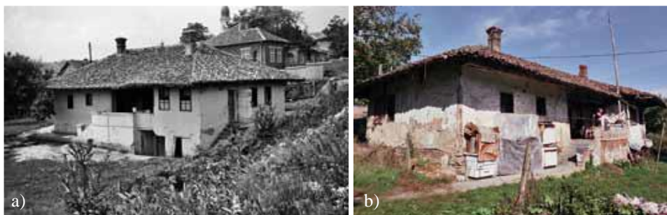
Fig. 4 Vljaković's house in Grocka: a) Appearance of the house in 1972 b) Current condition (Sources: M. Dedić, S. Negovanović)
