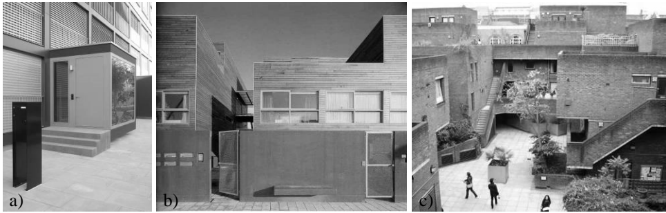
Fig. 4 a) Separated entrance to ground floor apartment directly from the public area; b) by means of private open space; c) separate entrances to apartments on lower floors above ground floor by means of separate access stairways
