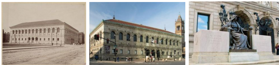
Fig. 1 Boston Public Library a) Old layout of the library [9], b) Renovated library, 2005 [10], c) Detail of "Bella Pratta" statue [11]
