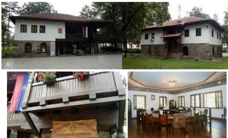
Fig. 2 Master Vasa's Residence in Kraljevo: a) Current condition of the exterior b) Spiritual center and working salon (Source: http://infokraljevo.com/gospodar-vasin-konak/ )
