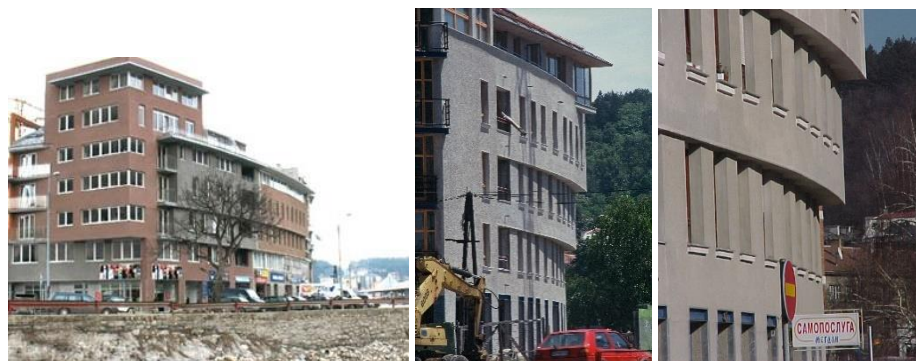
Figs. 9, 10, 11 Mixed-use buildings in Omladinska Street
