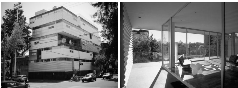
Fig. 3 Alfonso Reyes 58 apartment building (2003), Mexico City, Mexico / Dellekamp Arq.
