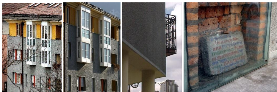
Figs. 5, 6, 7, 8 Architectural details showing the new blending with the old
