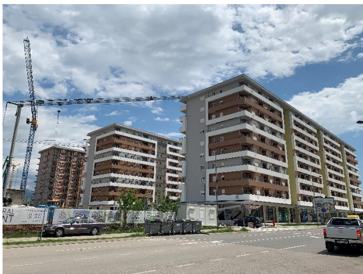
Fig. 5 “Central Point” – under construction (Source: personal collection)
