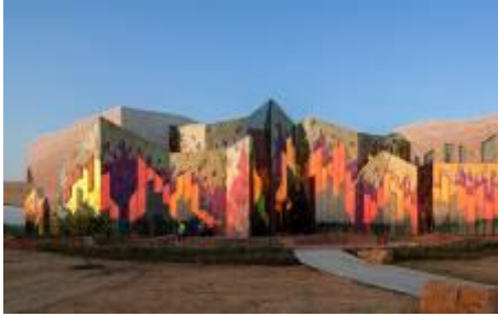
Fig. 11 The facade of the museum
