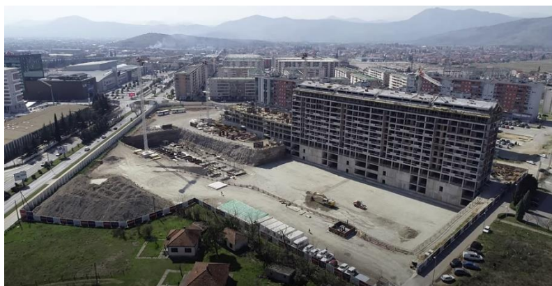
Fig. 6 “Master Quart” – under construction (Source: https://www.youtube.com/watch?v=Odos3utXmTI )
