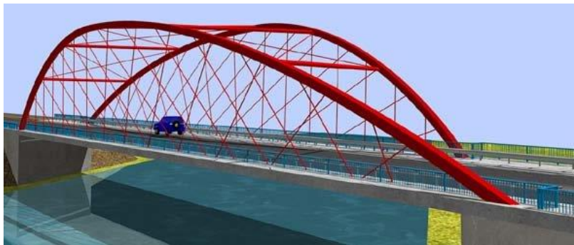
Fig. 4 Net-arch bridge with rolled I-sections in Poland (WD-57 Bridge)
