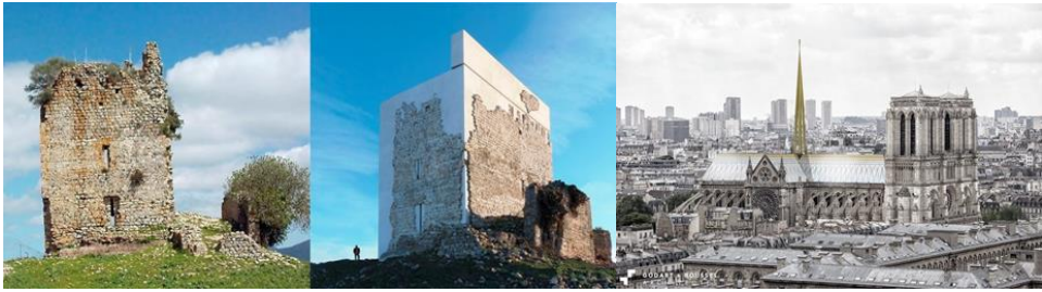
Fig. 1 a) Castle of Matrera before and after the restoration, b) One of the proposals for Notre Dame's reconstruction
