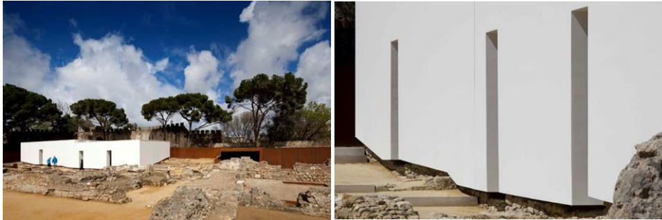
Fig. 6 A hovering protecting new structure
