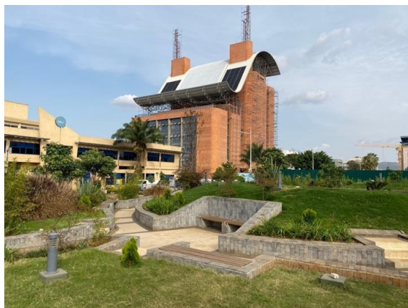
Fig. 1 I&M Bank HQ under construction © Ilija Gubić
