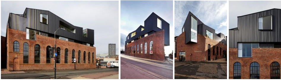
Fig. 2 The old brick house with a contemporary addition
