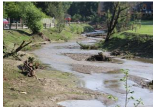
B. Widening the stream bed in the area of the Gasthof Pflieger. http://www.freiland.at/de/hws_schoeckelbach/
