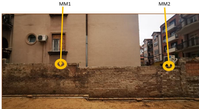
Fig. 5 Photograph of the wall separating the plot of the business building and the plot of the neighboring residential building; the positions of the measuring locations places are marked (view from the side of the office building)
