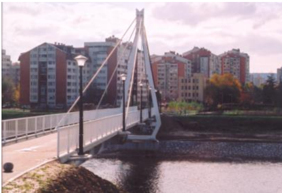
a) bridge view from the right river bank
