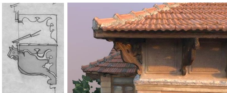
Fig. 3 Eaves detail - griffin, (left) drawing A. Blatnik, 1989, (right) photogrammetry A. Nikšić, 2020, [2]
