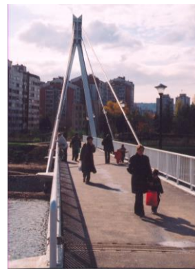
b) traffic on the bridge
