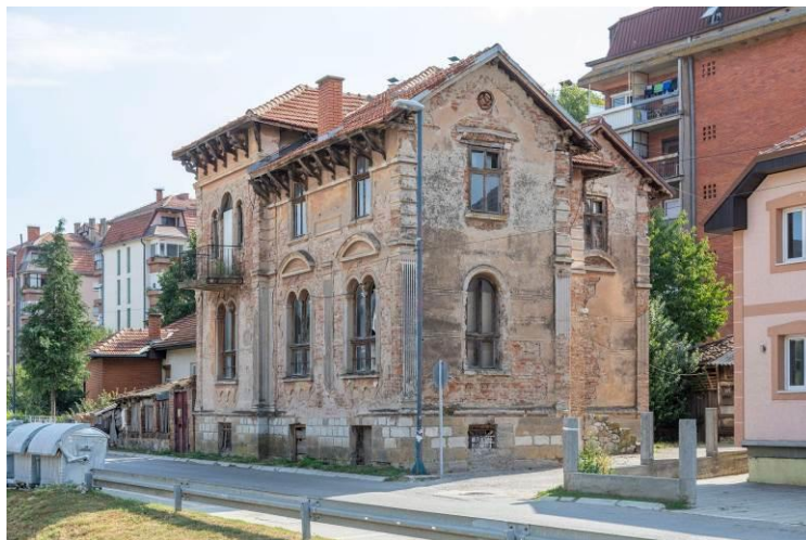
Fig. 2 Džadža's building in Dimitrovgrad, (photo Z. Radosavljević) [2]
