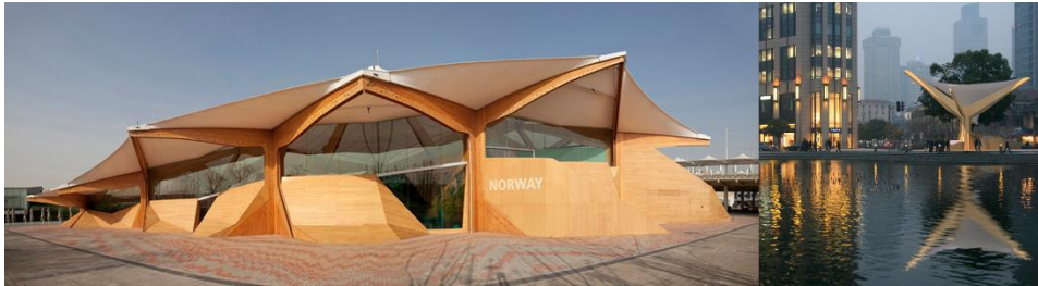
Fig. 9 Norway Pavilion in Shanghai 2010. [www.archdaily.com]
