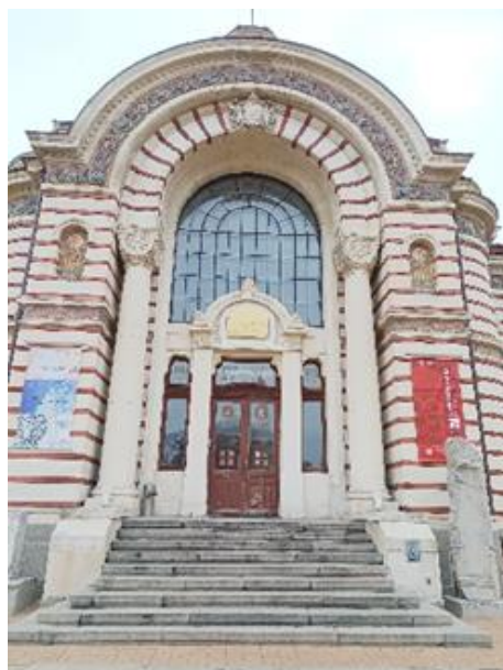
Fig. 8 The Central Mineral bath, detail from the façade, Sofia, 1907-1915, architect Petko Momchilov. Photography: Blagovesta Ivanova.
