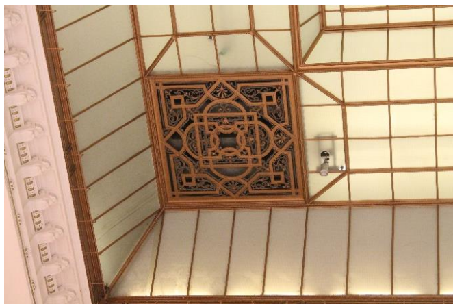
Fig. 4 Bon Marche, interior, Paris, 1876, engineer Alexandre-Gustave Eiffel and architect Louis-Auguste Boileau. Photography: Blagovesta Ivanova.
