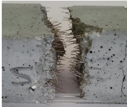
Fig. 3 Appearance of the concrete with steel microfibers at the failure point after testing the flexural strength
