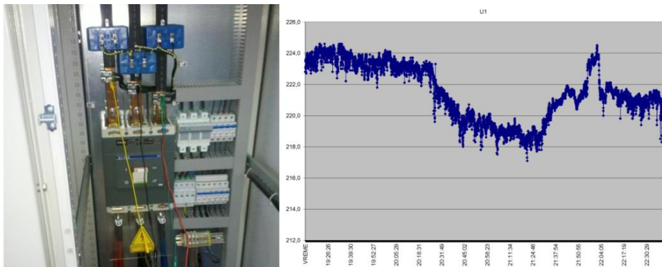
Fig. 3 Continual measurement of the phase voltage using the VMP20 instrument.
