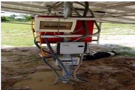
**Fig. 13** Pump controller
