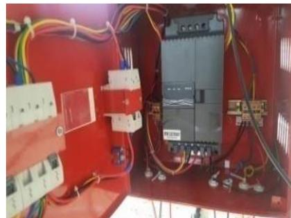
**Fig. 14** Variable frequency drive
