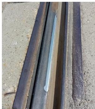
**Fig. 3** Austenitic layer in the rail surface
