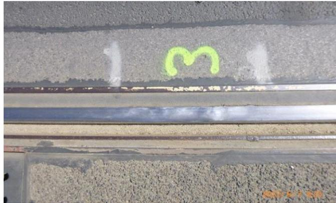
**Fig. 6** Wear on the running surface at a welding in paved track
