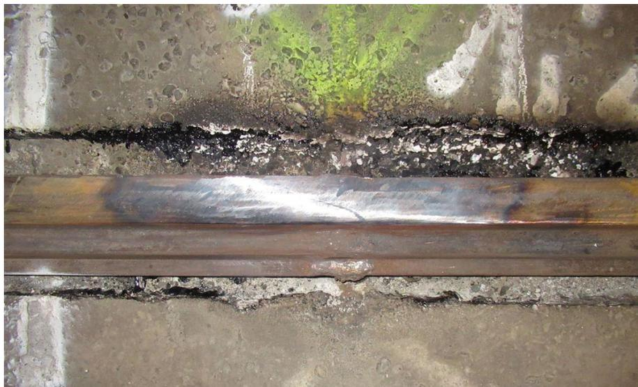
**Fig. 13** Partial preheating on the selected location
