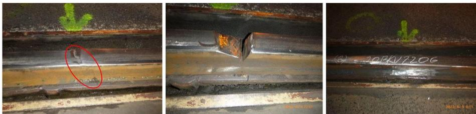
**Fig. 11** Welding of a rail crack (left – crack, middle – preparing, right – completed welding)
