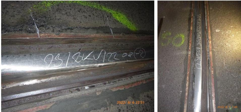
**Fig. 8** The completed welding after grinding
