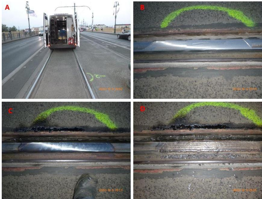
**Fig. 7** Technology steps. A – removed embedding pouring next to the rail head, B – preparing the surface, C – preheating, D – welding
