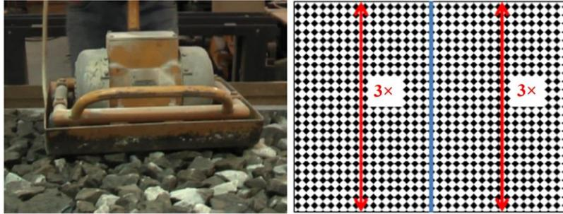
**Fig. 4** Vibrator compaction tool and compaction processions
