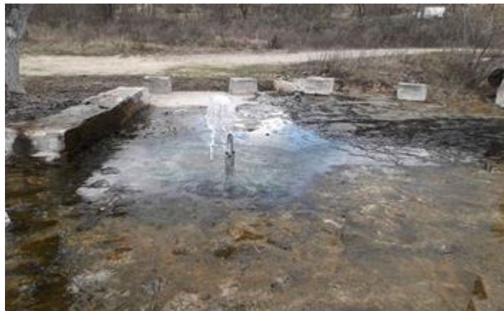
Fig. 2 Water bursting in Spring 1 in Tulare
