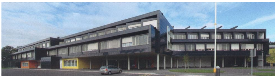
Fig. 7 The Ljubljana Conservatory for Music and Ballet in the new building where the lessons began in the school year 2008/2009
