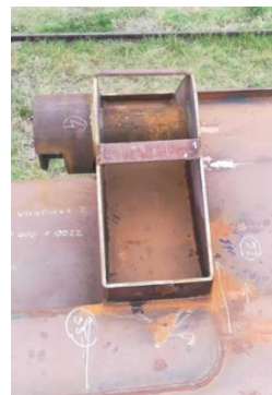
Fig. 1 Steel support No.4 of the harbor pontoon access bridge
