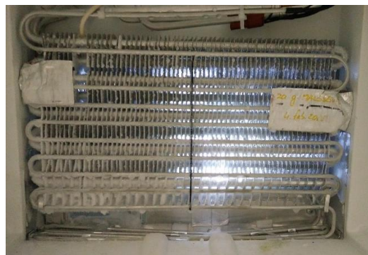
Fig. 3 Rime and clear ice on the evaporator
