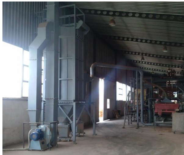
Fig. 3 Layout of the filter system applied to the system for the preparation of bituminous materials for road construction
