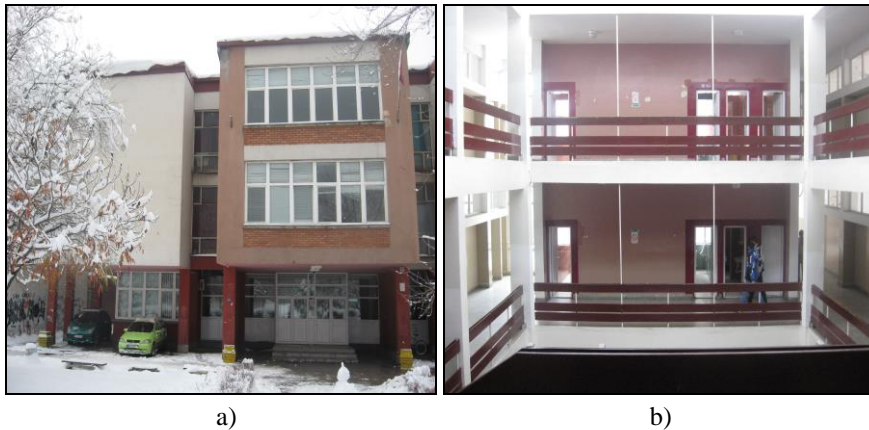
Fig. 3 Electrotechnical School “Nikola Tesla” in Niš - front side (a) and the hall in classrooms part - inside (b)
